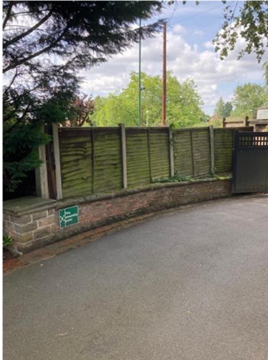
Vehicle Exit Gate.
