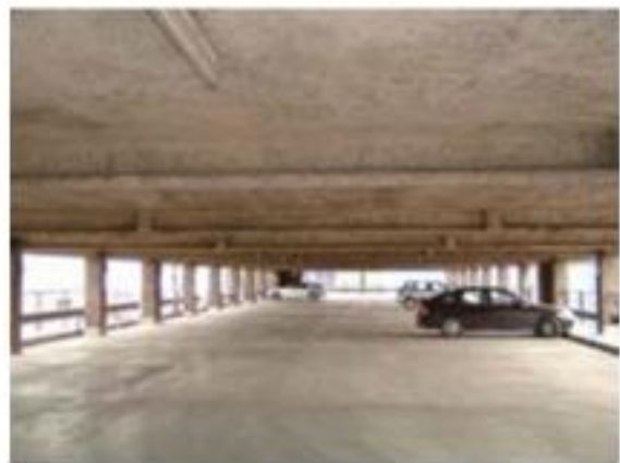
Sprayed asbestos fire protection on concrete structures
