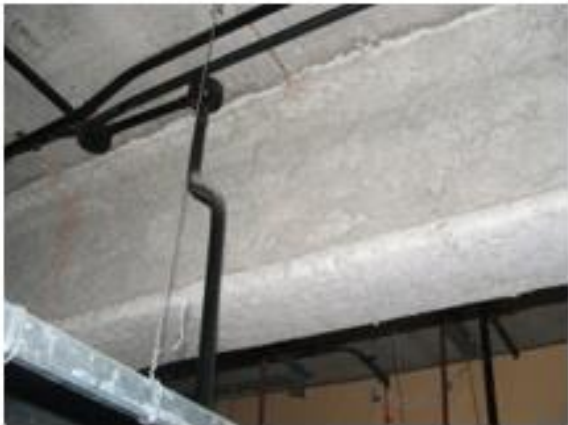
Sprayed finish on beams in ceiling void
