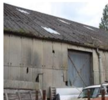
Asbestos sheeting and downpipes
